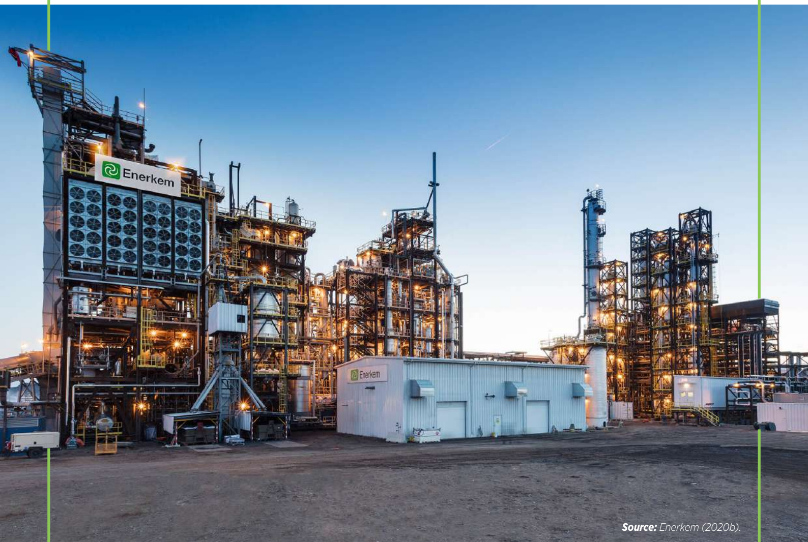
Figure 21. Enerkem’s MSW to biofuels (methanol and ethanol) plant in Alberta, Canada.
